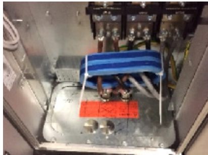
Fig. 6.21 Common-mode cores installed at the drive terminals
